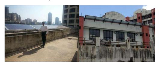
Structure on parafait wall with support from outside wall of the building
